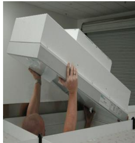
Figure 4: FFU pushed up on one side for removal
