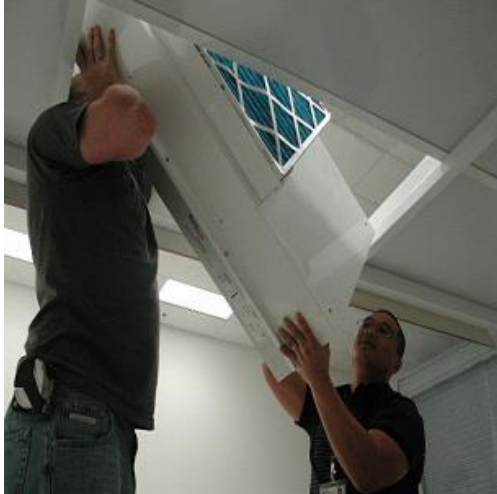
Figure 5: Personnel rotating FFU to remove from ceiling grid
