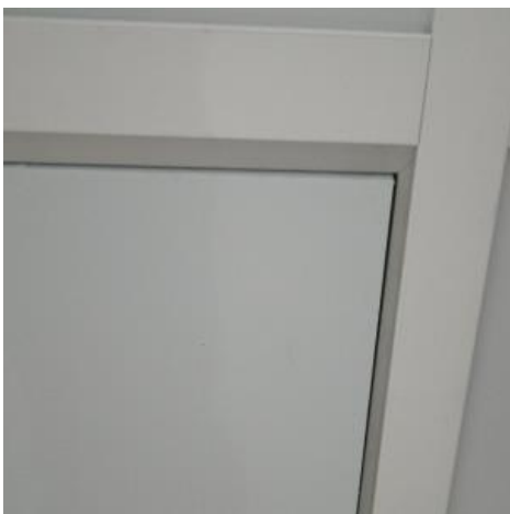
Figure 3: Panel fully attached to filter screen without overlapping edges
